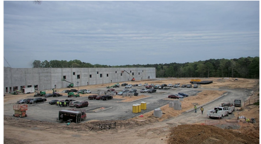
Durham Coca-Cola Bottling Company Headquarters progress, April 2024
